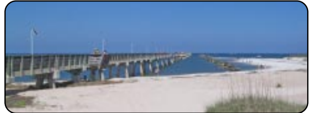
The Fort Clinch Fishing Pier is nearly a mile long.
