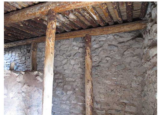
Details of room structure
